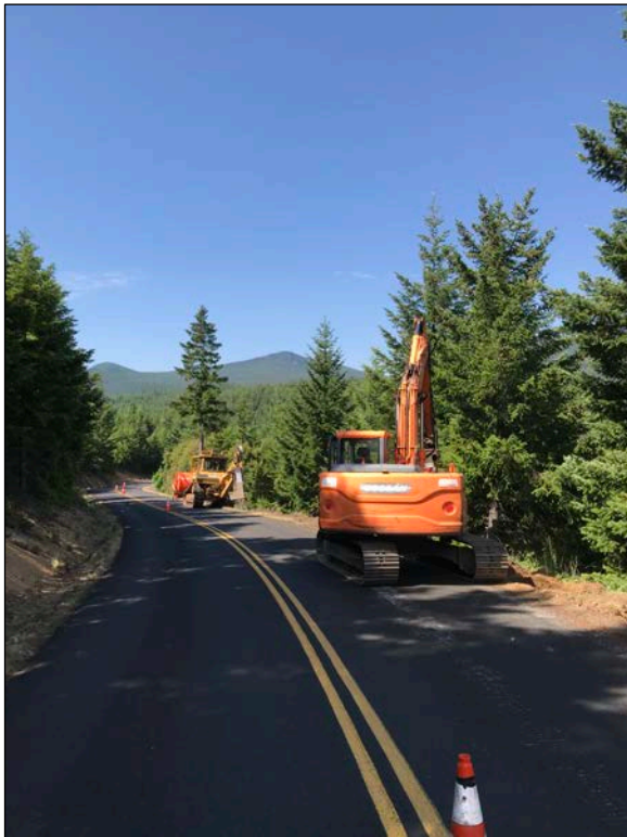
Photograph 2. Example of a running line installation using the trenching method on the highway shoulder. Photograph taken on a different Zayo fiber optic project.
