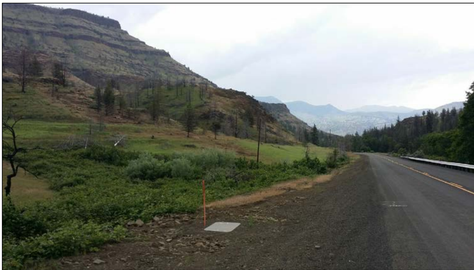
Photograph 4. Example of a vault/handhold located adjacent to the road prism, as shown by the orange marker. Photograph taken in a newly constructed portion of the project.
